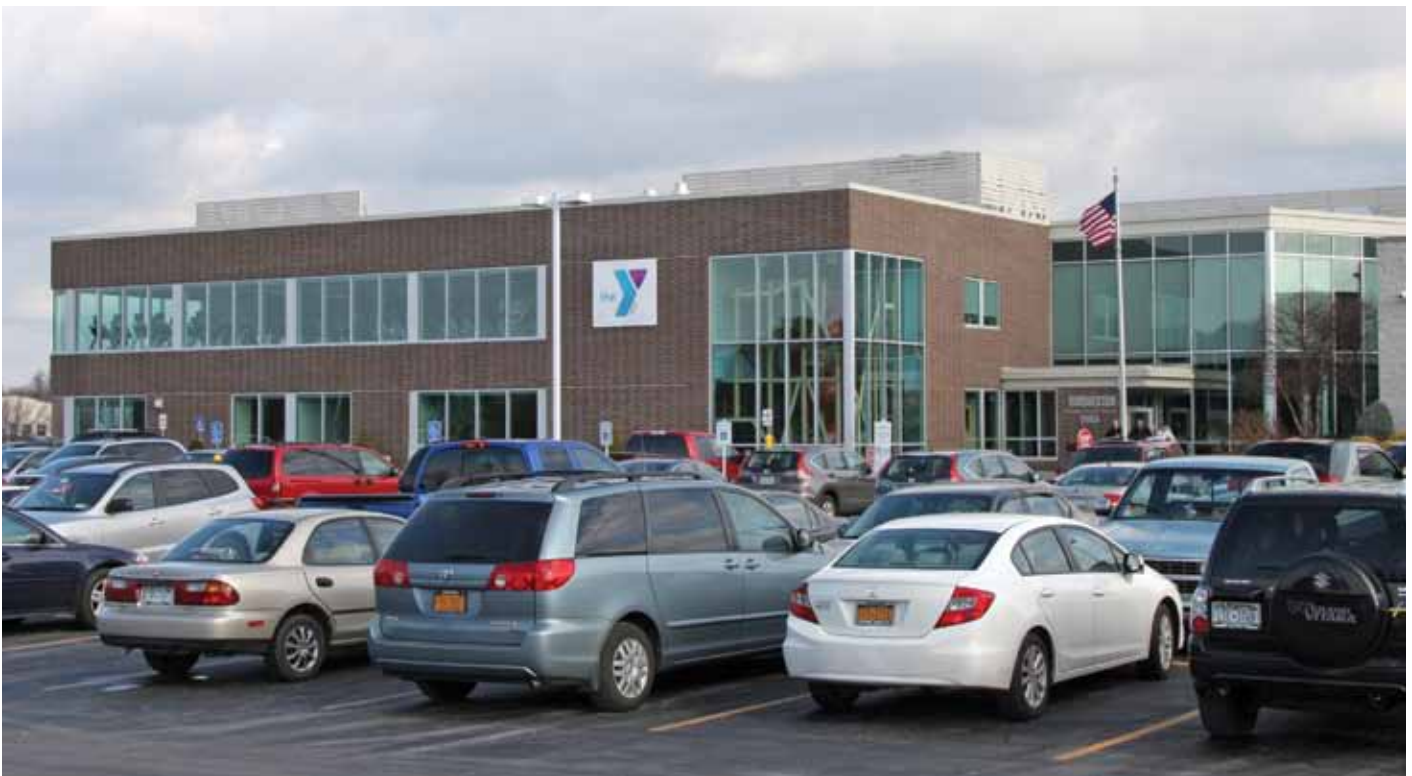
View of Westside Family YMCA
