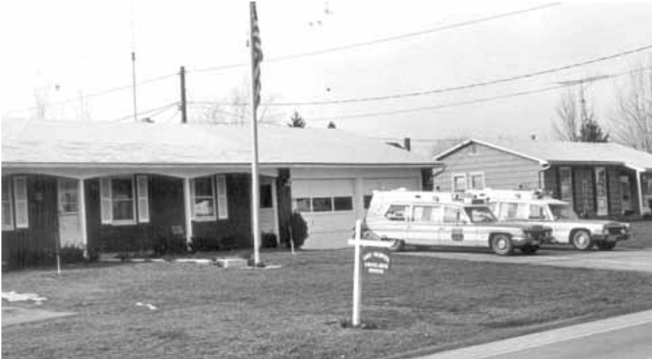
The headquarters at 144 Gatewood Avenue was opened on June 18, 1966. The original garage opened onto Gatewood Avenue. A single-bay garage opening onto Howard Road was added during the first remodeling project. A second bay facing Howard Road was added a few years later, as seen in this photograph.
