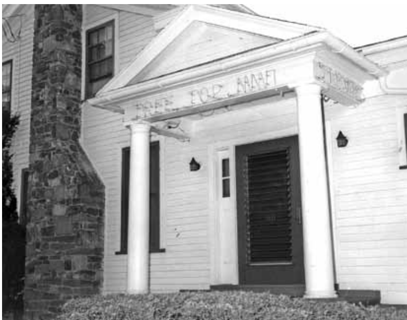
Steve's Tree Top Inn —Steve's Tree Top Inn on the corner of Long Pond Road and Spencerport Road was a favorite local restaurant and bar.
