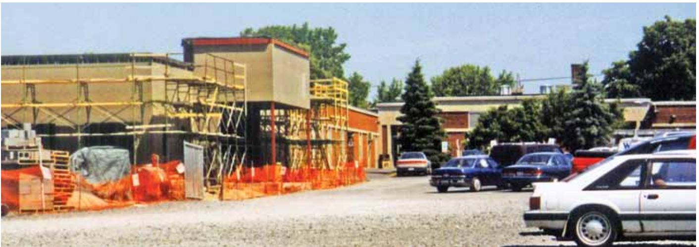
Gates Town Court Addition —The Gates Town Court addition to the Community Center is pictured during construction circa 1999. The previous court facility in the Town Hall regularly had overflow crowds as the case load for the Gates town courts grew beyond the capacity of the 1969 court room.
