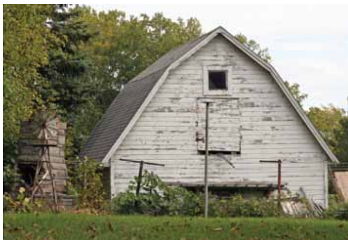
Gates Barn Near Lee Road and Trolley Boulevard with Unusual Hip Roof Style
