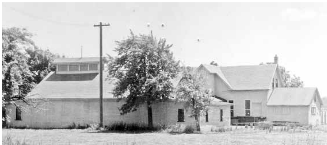
John Kuhn Home —This was the Lyell Avenue residence of John Kuhn, pictured on June 7, 1960. It, too, was razed for construction of Interstate 390. Many other Gates homes and streets were also removed for this expressway. Note the lack of homes on the east side of Beechwood Drive and the west side of Evelyn Drive. These homes too were removed to make way for the Outer Loop.
