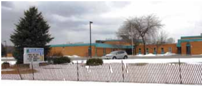
Exterior of Walt Disney School 2013
