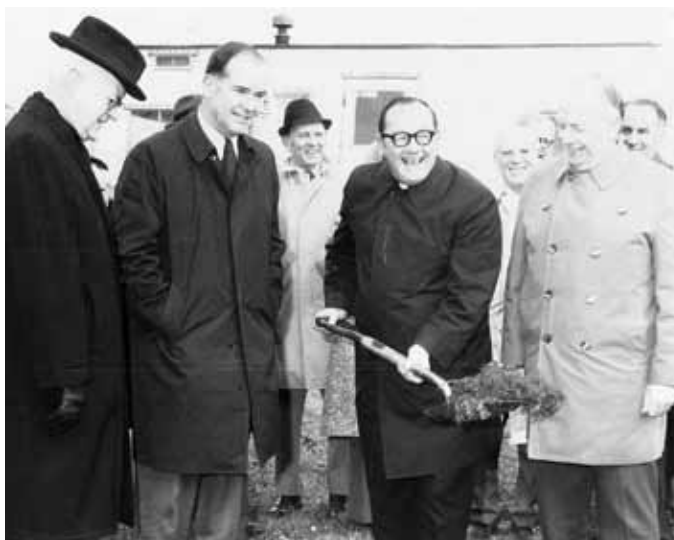
Groundbreaking for Dunn Tower I, December 1, 1973. Among those identified in the photo are (left to right): Monsignor Reverend Dennis Hickey; Congressman Barber B. Conable Jr.; Gates Councilman James O'Neil; the Reverend Gerald E. Dunn, holding the shovel; Frank Bott; Albert Hinkle, assistant commissioner of the New York State Division of Housing and Community Renewal; and Gates Councilman John Maggio.
