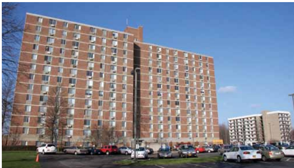
View of the two towers
