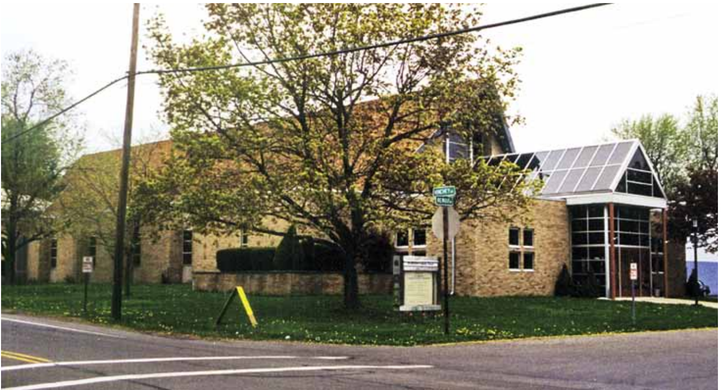
View of St. Helen Church, 310 Hinchey Road
