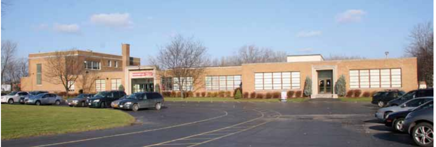
View of Northstar Christian Academy, formerly the Warren Harding elementary school for Gates Chili School District
