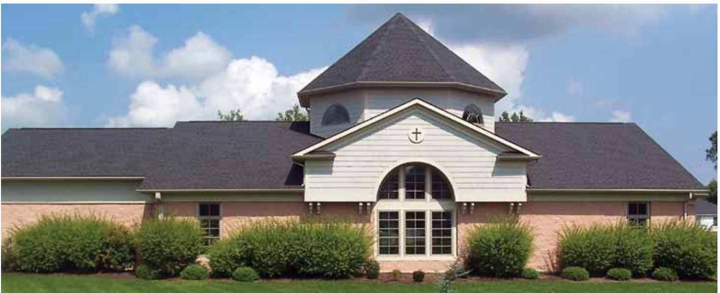
Front view of St. Nicholas Church
