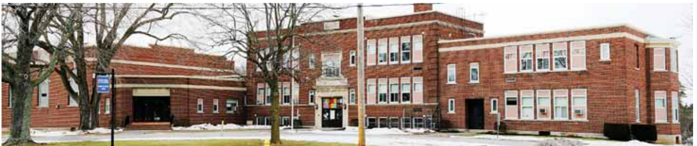
Exterior of Washington Irving School on Chili Avenue, now rented to Generations, a for profit day care and elder care facility
