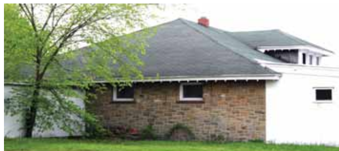
Becker's Adapted Barn on Buffalo Road —Some barns have been modified into other uses and are no longer recognizable as barns. Pictured here is the original carriage barn of the former Gates Presbyterian Church. The barn has been adapted for modern use as a part of Becker's Furniture on Buffalo Road just east of Howard Road. During church services in its day, the carriages that transported churchgoers were stored in this stone building. Visitors can clearly see the original stone walls when visiting the adjacent Gates Cemetery.
