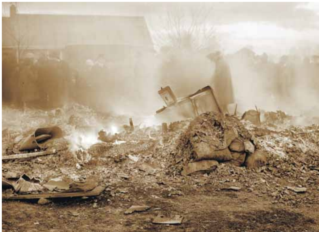
Two children died in this house fire on Evelyn Street on November 19, 1923. The photograph was taken by Albert R. Stone, Rochester's first photo-journalist, and appeared in The Rochester Herald newspaper the next day. Firefighters from the city of Rochester, neighbors, and onlookers appear as ghostly images through the smoldering ashes. A few hot spots can also be seen.
