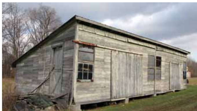
Coldwater Road Shed
