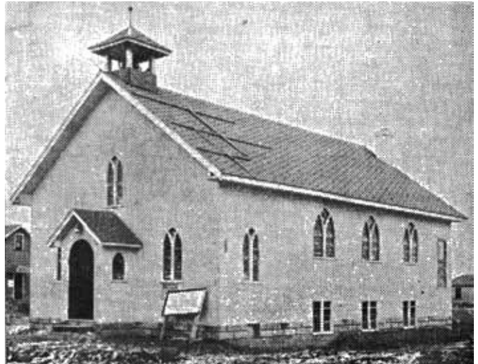
Original church under construction
