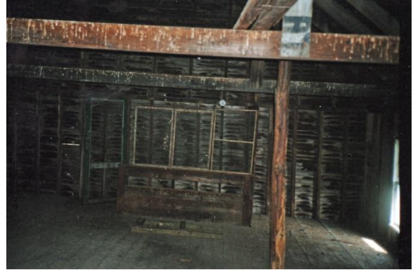
Figure 4: barn 3rd floor shows use of old railroad boxcars
