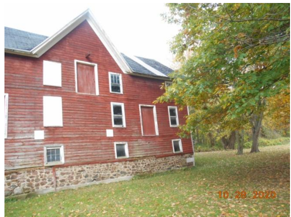
Figure 5 : barn south side today
